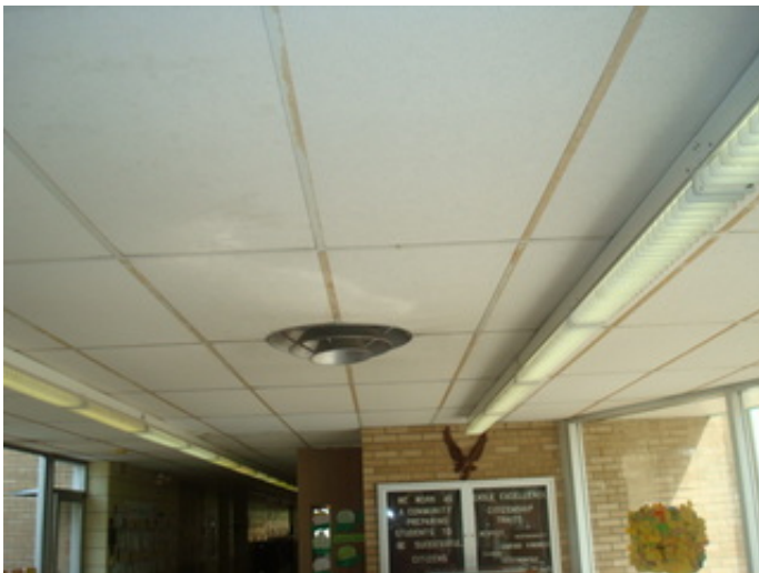
Ceiling without fire suppression
