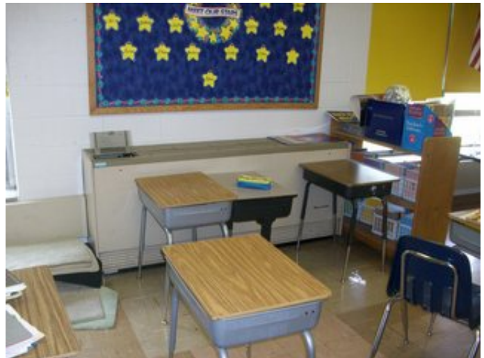
Typical Room Unit Ventilator
