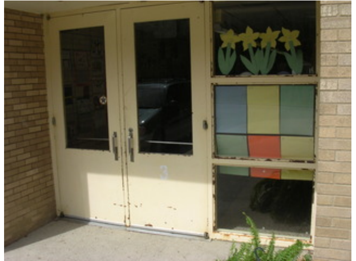
Typical hollow metal entry doors.
