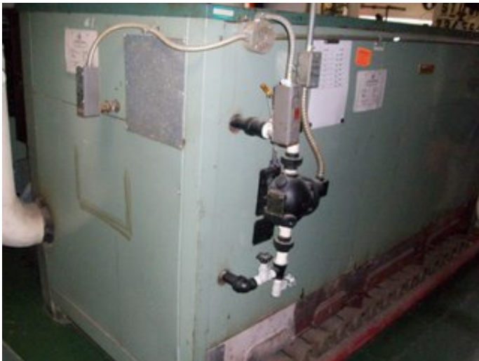
Gas Fire Hot Water Boilers
