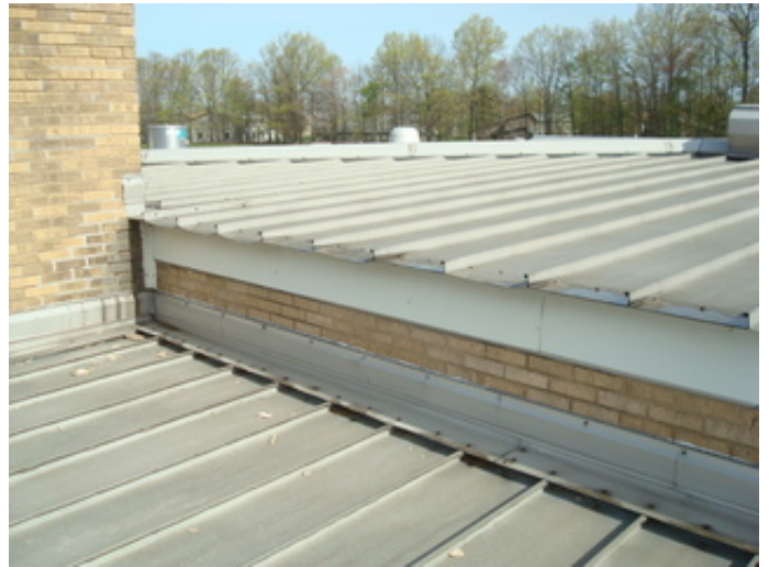
Metal roof flashings
