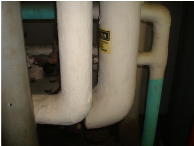
Pipe fittings and insulation
