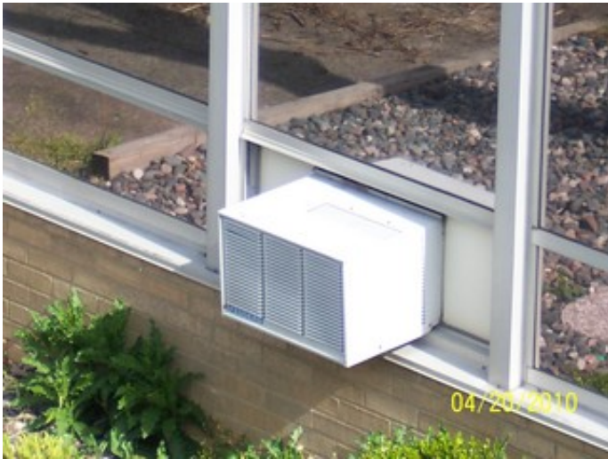
Typical Window Air Conditioner Unit
