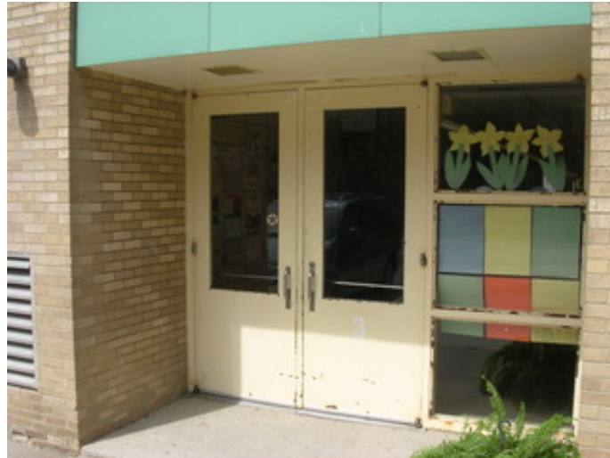
Typical hollow metal storefront system.
