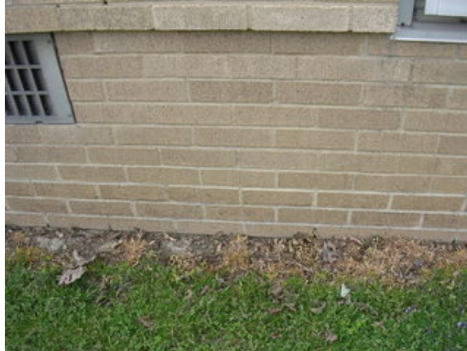
Typical foundation condition.
