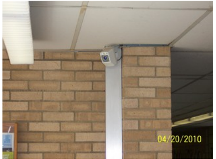
Main Entrance Security CCTV Camera
