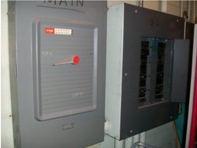
Main Electrical Switch & Distribution Panel
