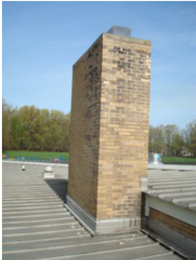
Chimney with damaged brick
