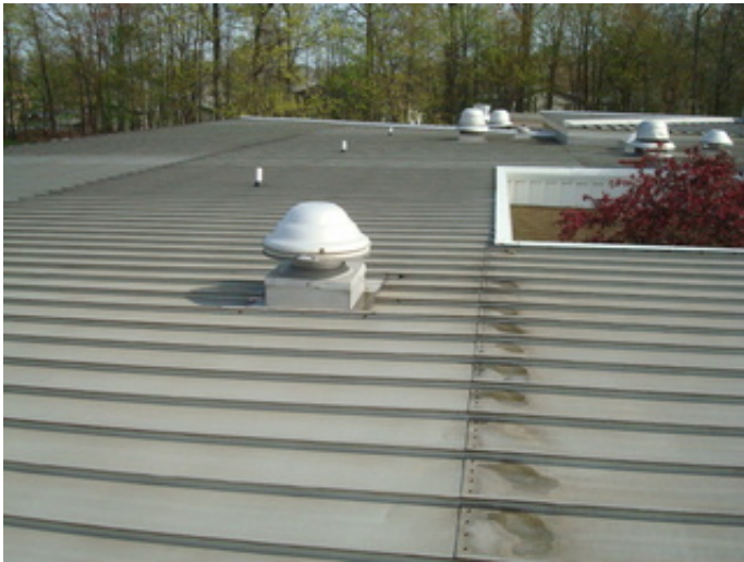
Metal roofing seam
