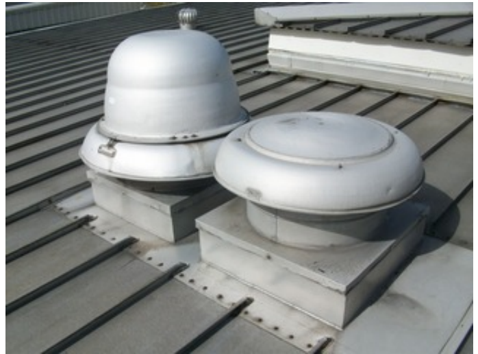
Roof Mounted Exhaust Fans
