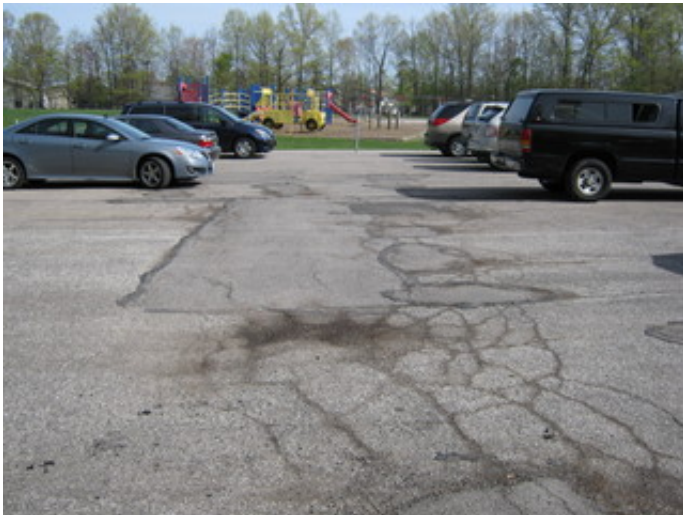
Parking lot in poor condition
