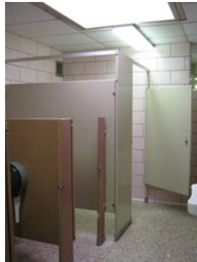
Compliant toilet stall
