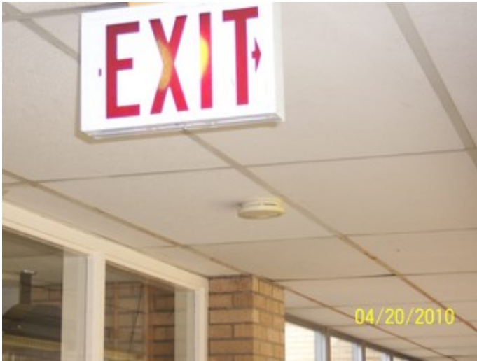
Typical Exit Sign
