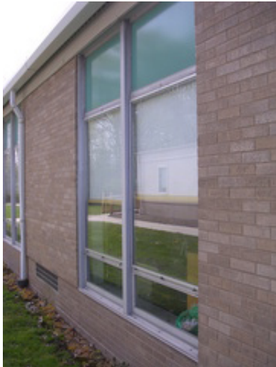
Typical aluminum window system.
