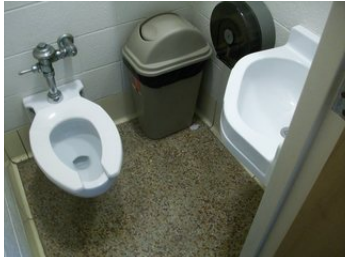
Toilet room fixtures
