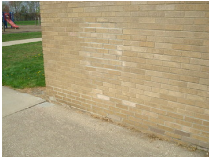
Damaged brick with insufficient weep holes
