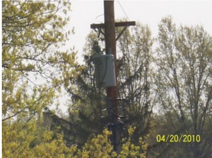
Pole Mounted Transformer
