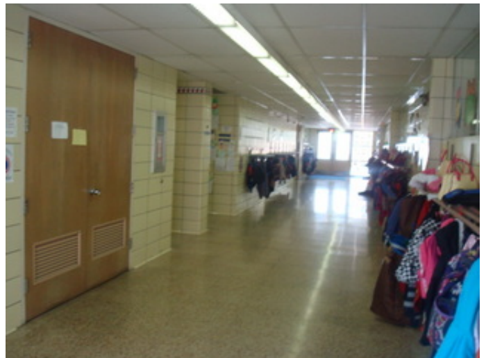
Corridor with fire extinguisher cabinet
