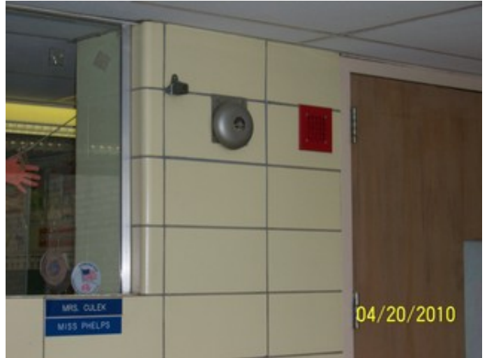
Typical Fire Alarm Devices
