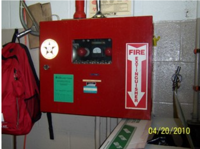
Main Fire Alarm Panel
